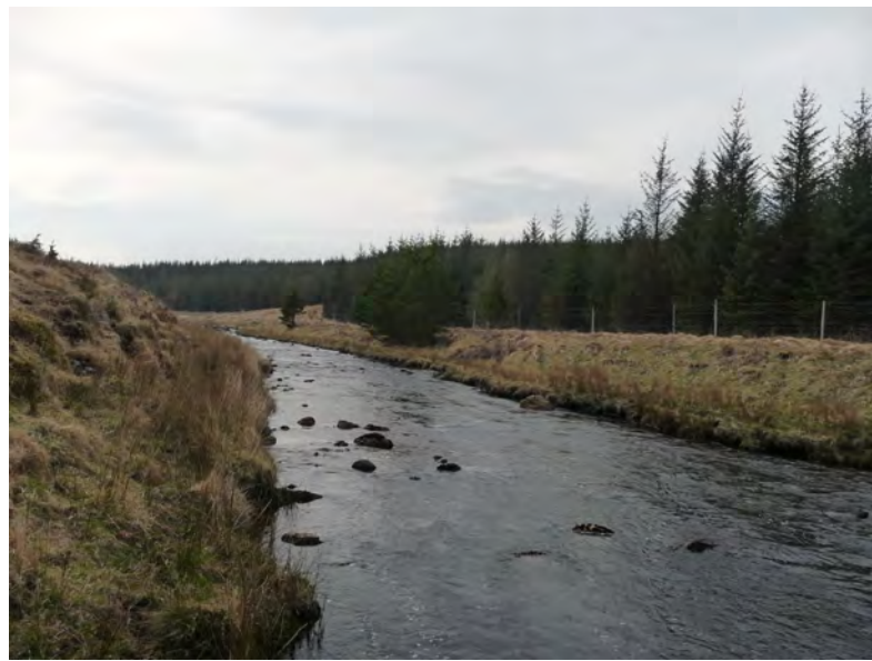
WATERCOURSE CROSSING 3 - VIEW UPSTREAM
