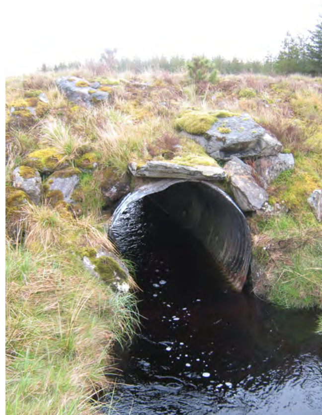
WATERCOURSE CROSSING 7 - CULVERT
