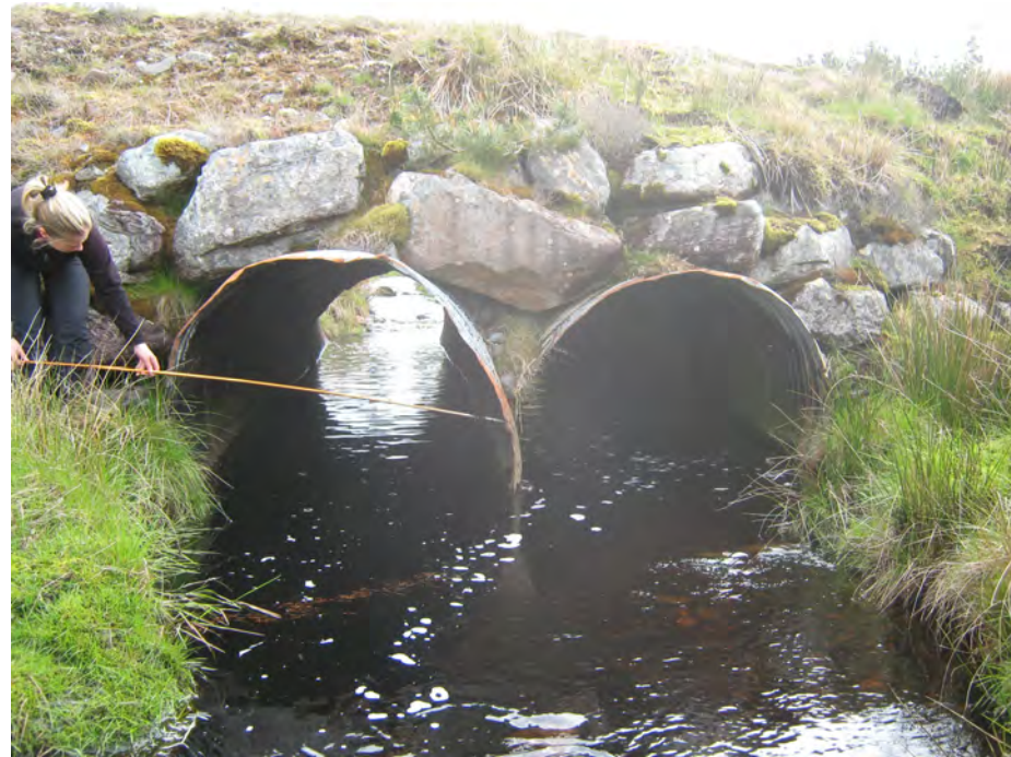
WATERCOURSE CROSSING 16 - VIEW UPSTREAM
