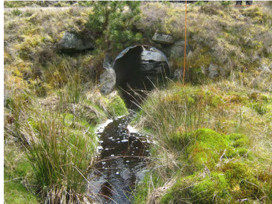
WATERCOURSE CROSSING 9 - VIEW UPSTREAM
