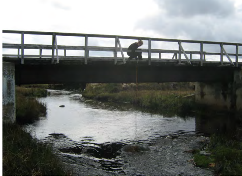
WATERCOURSE CROSSING 5 - VIEW UPSTREAM
