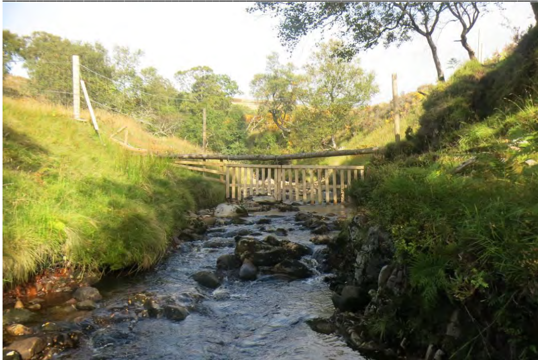
Figure 31: One of three water gates within channel – fully accessible to fish
