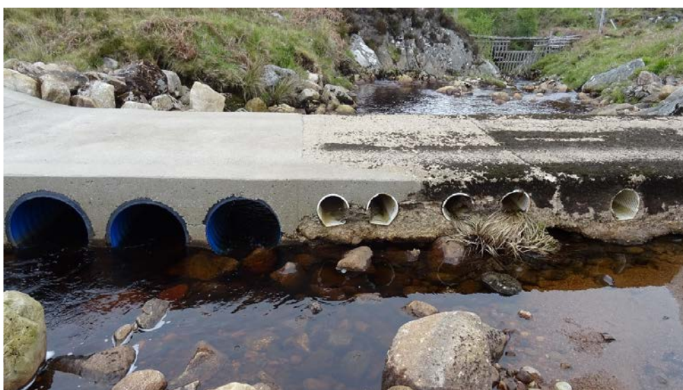
Photograph A9.2: Existing Crossing of the Allt a' Mhuilinn (Looking Downstream)
