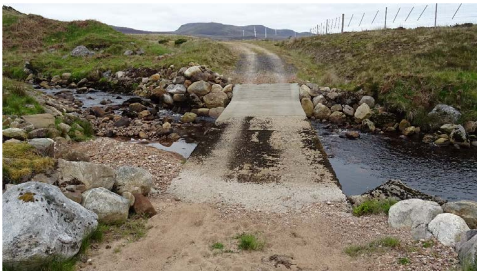
Photograph A9.1: Existing Crossing of the Allt a' Mhuilinn
