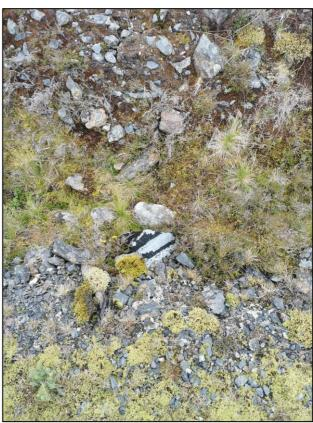
Example of existing pipe with insufficient cover and deformation
