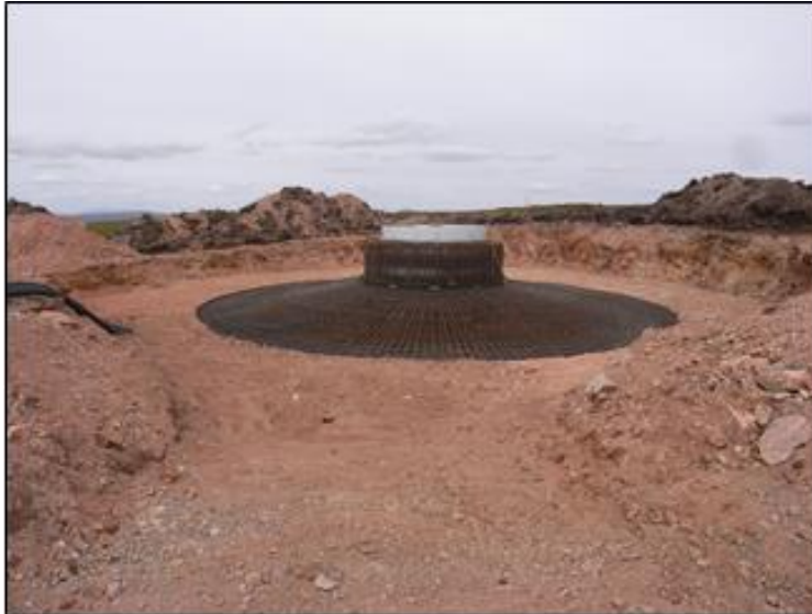
Plate 4.1: Construction of Turbine Foundations (photos from Gordonbush Wind Farm)
