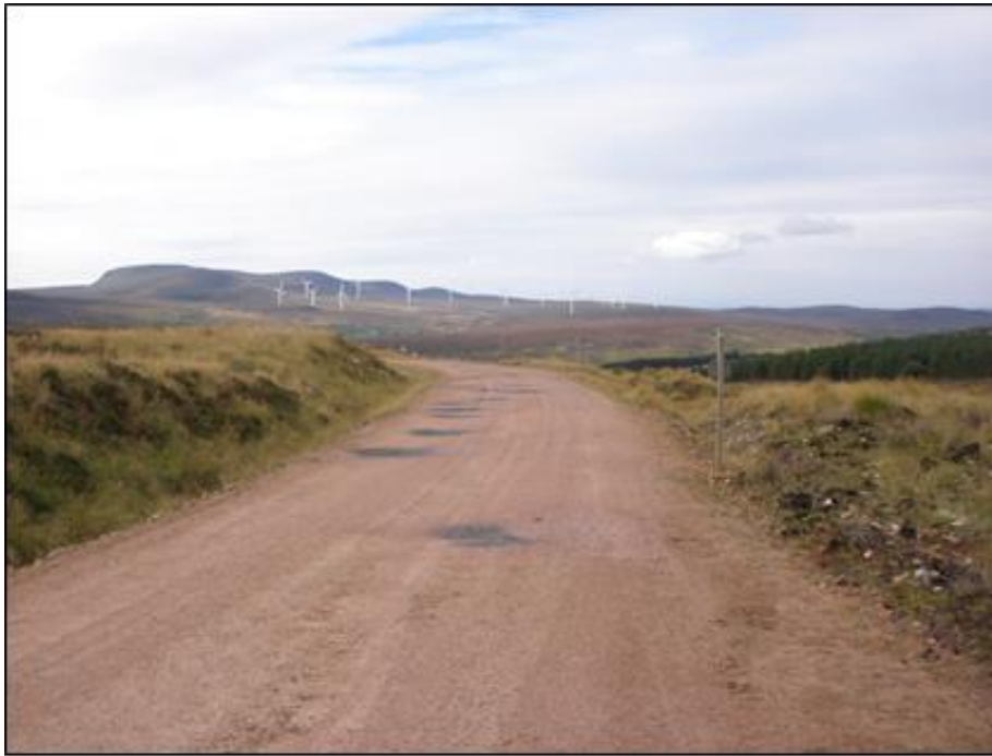
Plate 4.2b: Existing Gordonbush Wind Farm Access Track
