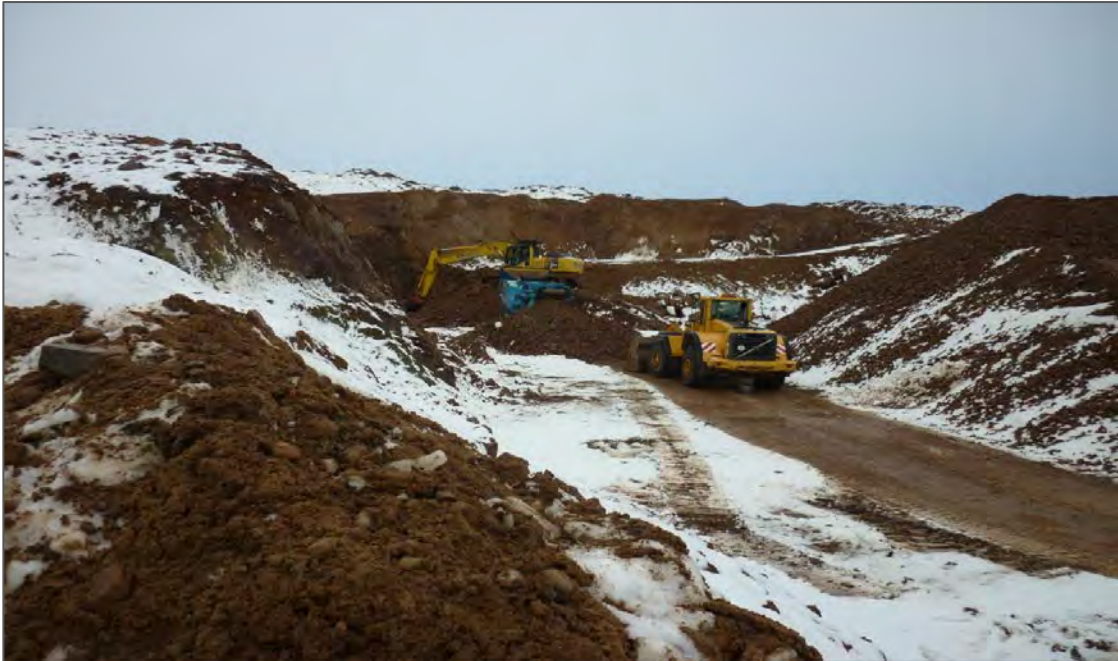
Photo 3--3 Borrow Pit BP1 in operational stage showing vertical high wall.
