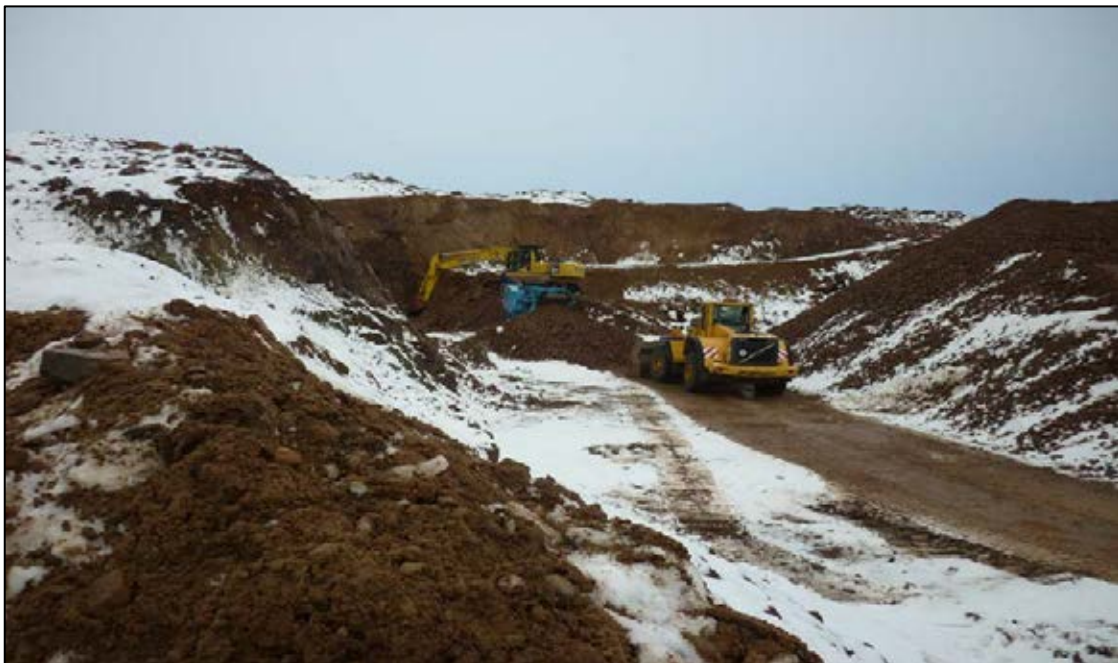
Photo 3 – Borrow Pit BP1 in operational stage showing vertical high wall.
