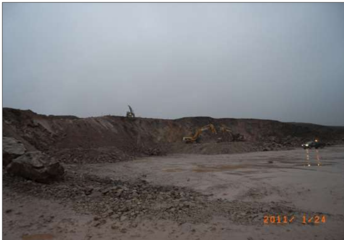
Photo 3-4 Borrow Pit BP2 in operational stage showing vertical high wall.
