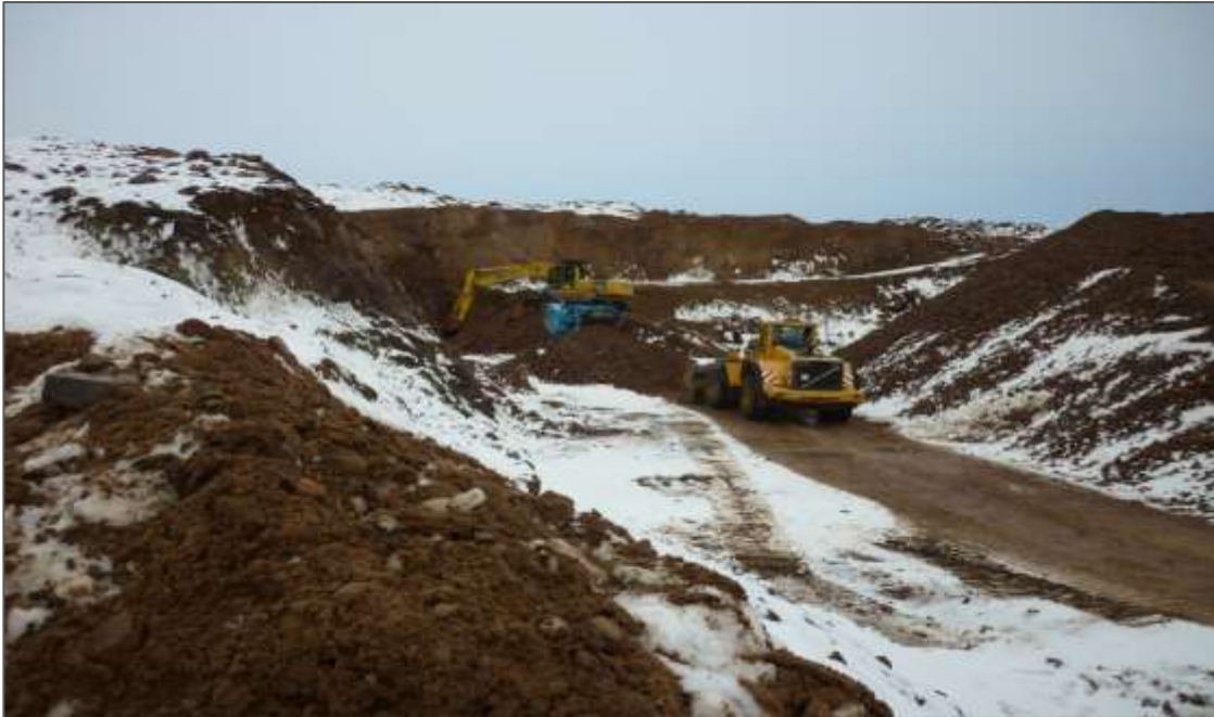
Photo 3-4 Borrow Pit BP2 in operational stage showing vertical high wall.
