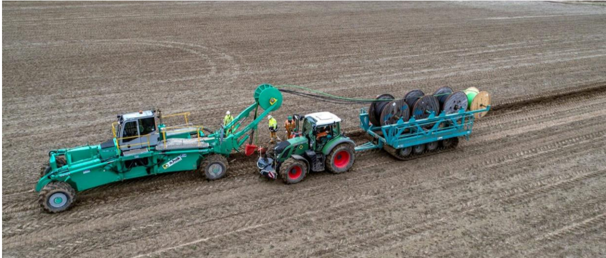
Plate 2: An example photo of cable ploughing
