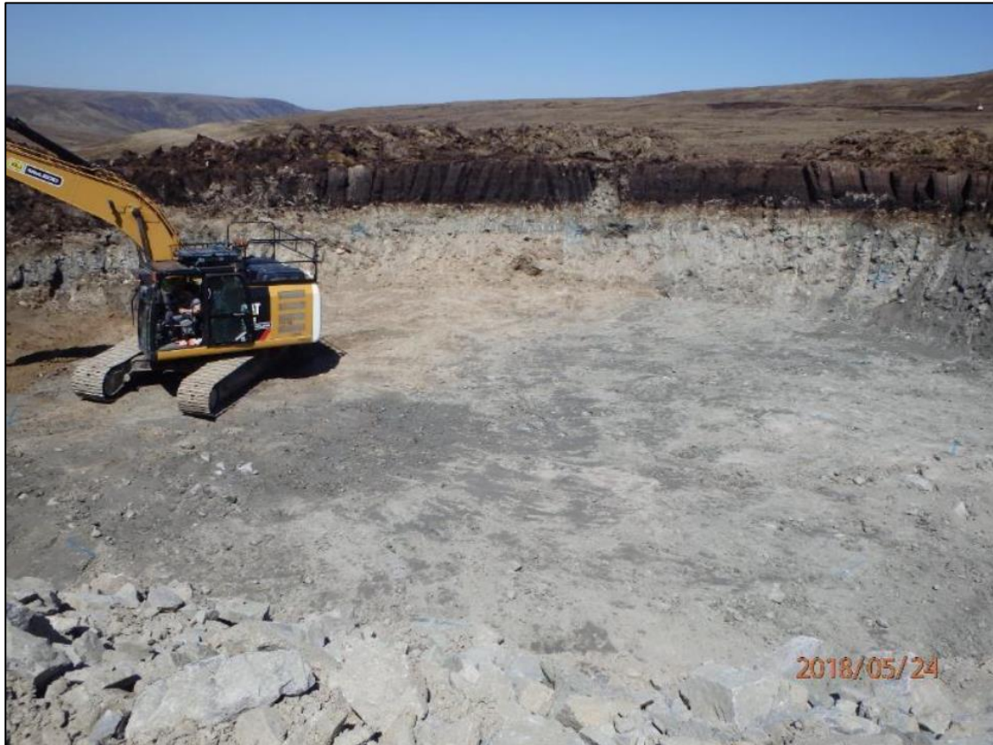
Plate 3.2: Example Turbine Foundation Construction – Excavation
