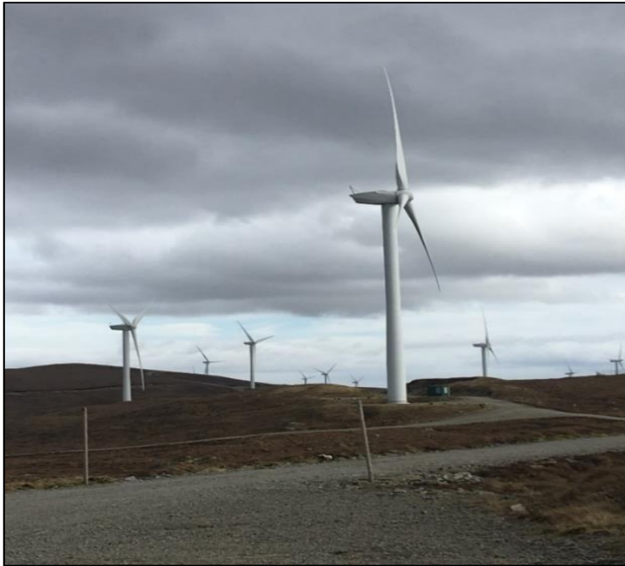
Plate 3.1: Existing Track Infrastructure, Achany Wind Farm
