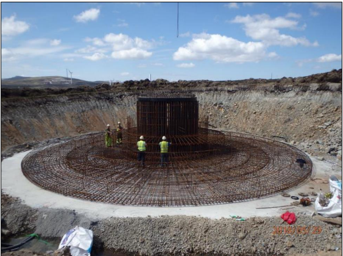
Plate 3.4: Turbine Foundation Construction – Steel Reinforcement
