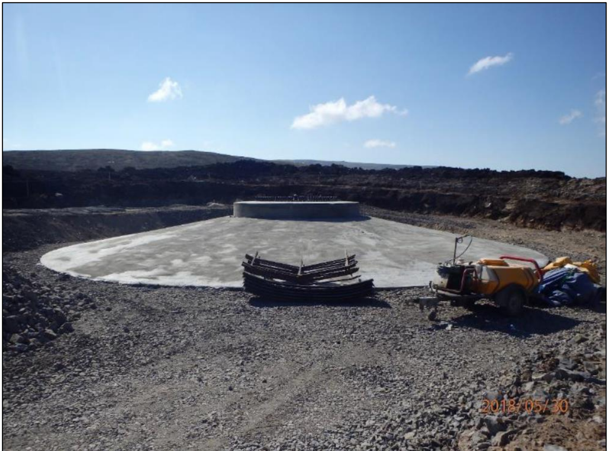
Plate 3.6: Turbine Foundation Construction – Completed Foundation (to be backfilled)
