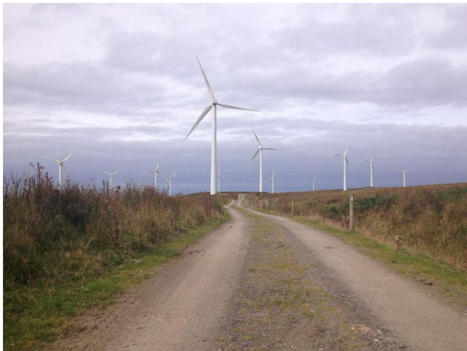
5.3.19 Depending on local ground conditions, access tracks will be constructed using either a 'floating track' or a 'cut track' design. Figure 5.1 shows the indicative locations of cut and floated track which will be refined post consent during the detailed design phase.
