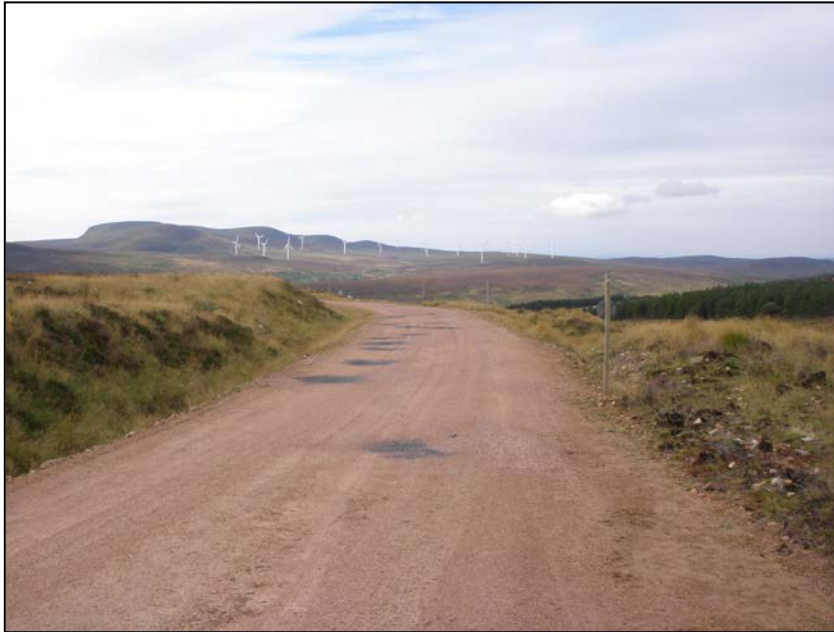
Plate 4.2b: Existing Gordonbush Wind Farm Access Track
