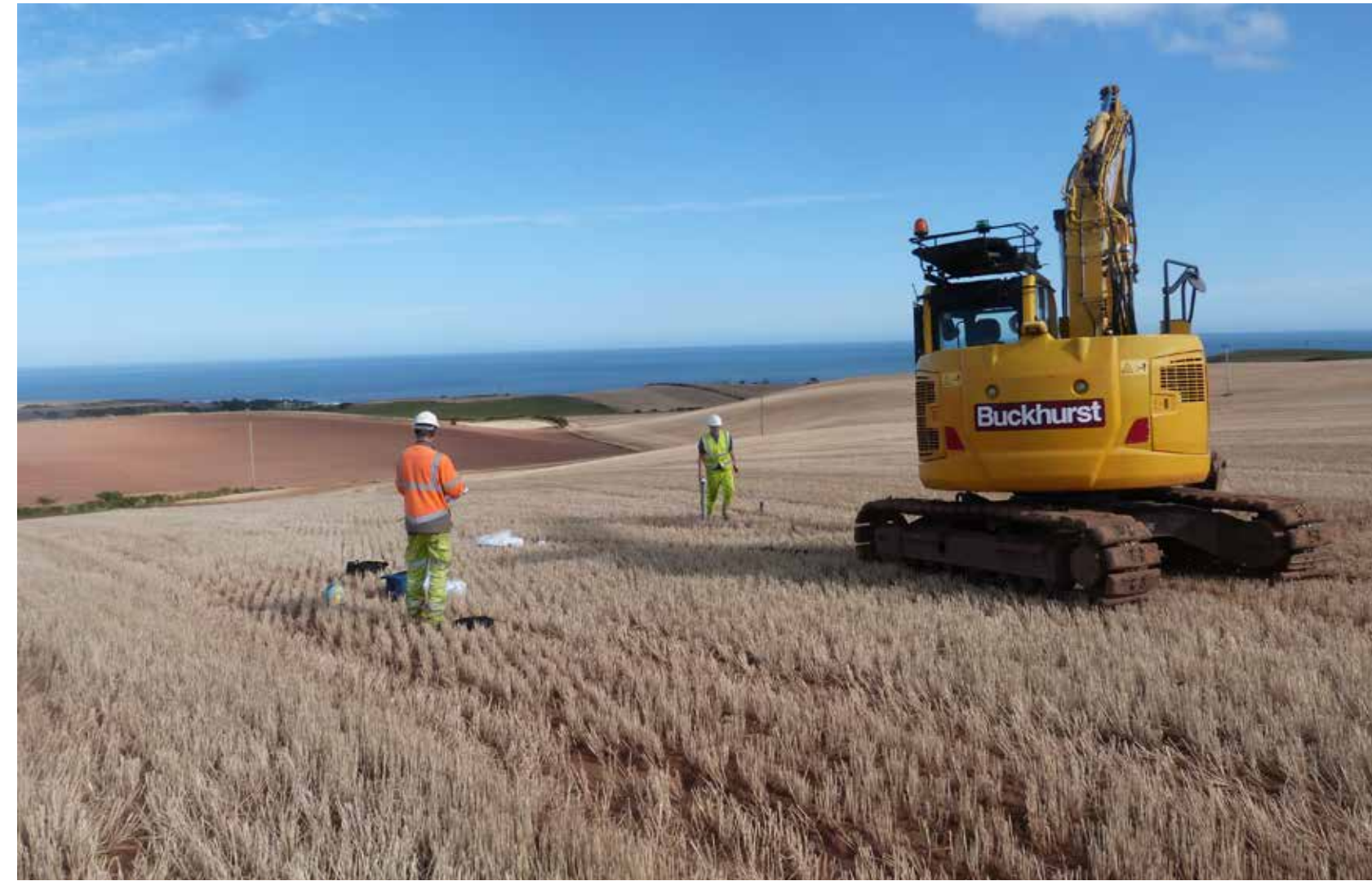
Ground investigation works
