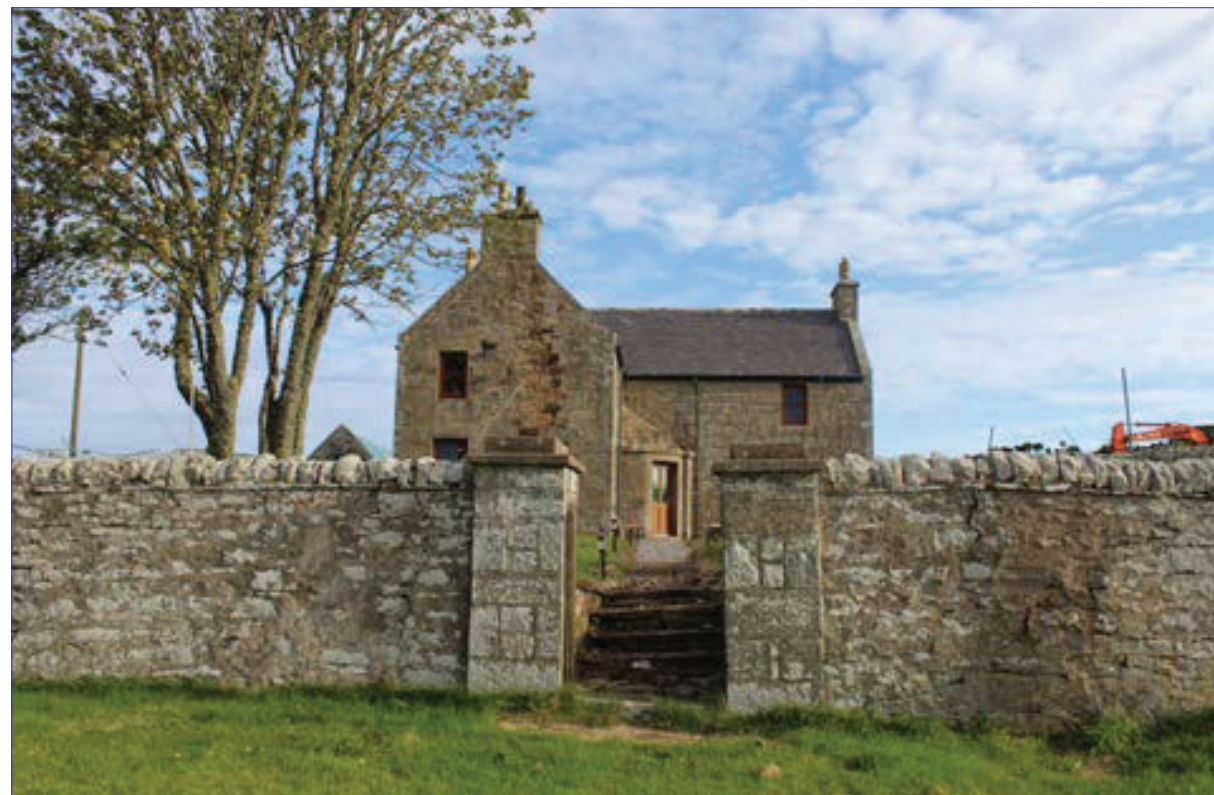
Plate 7.6: North facing view of the Category C Listed Strathy Former Manse (Site 24)
