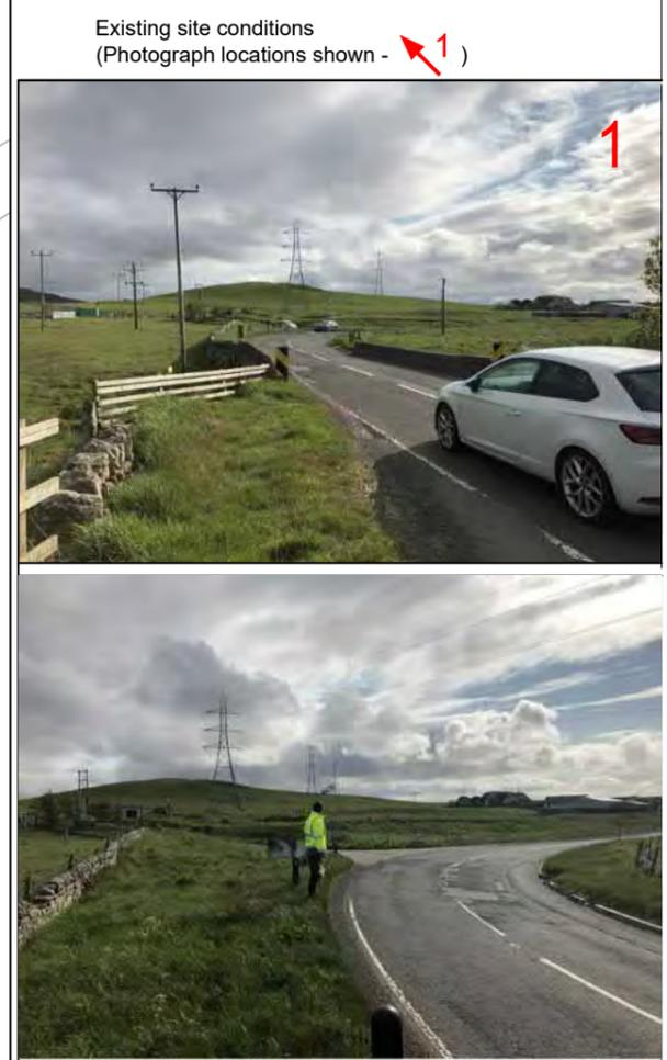
Temporary over-run of existing hard strip (footway) required to accommodate abnormal loads. Surface to be protected with heavy duty steel load bearing spreader plates for the entire duration of abnormal load delivery programme. In addition, temporary ramp to be formed with cold tar to be installed in front of kerb to allow abnormal load vehicles to mount the kerb without causing undue damage
