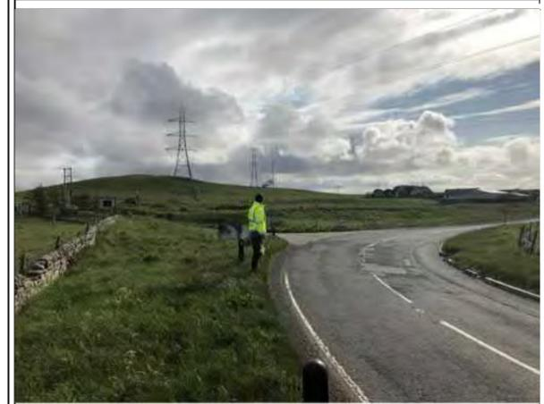
Temporary over-run of existing hard strip (footway) required to accommodate abnormal loads. Surface to be protected with heavy duty steel load bearing spreader plates for the entire duration of abnormal load delivery programme. In addition, temporary ramp to be formed with cold tar to be installed in front of kerb to allow abnormal load vehicles to mount the kerb without causing undue damage
