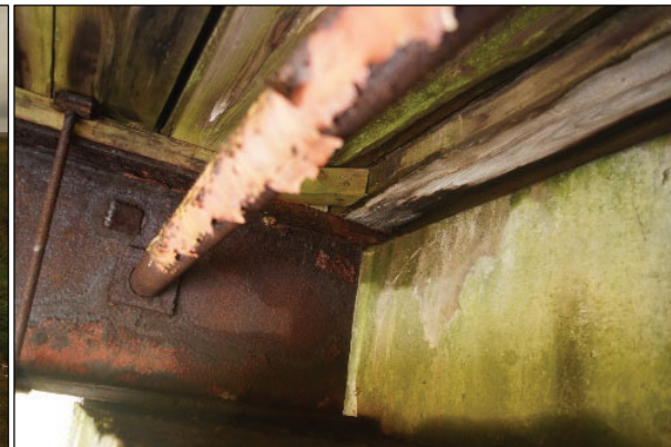
Photo 22. Small gaps exist but the bridge has low bat roost potential.
