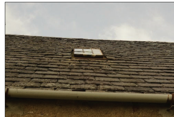
Photo 25. Potential roosting features are gaps under the roof slates and guttering (east aspect).
