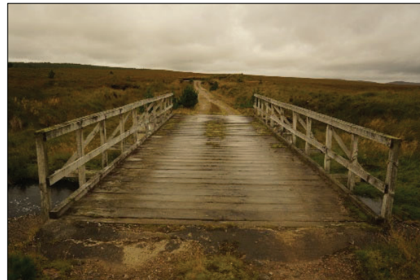
Photo 21. Strathy River Bridge spans Strathy River on the east of the site.
