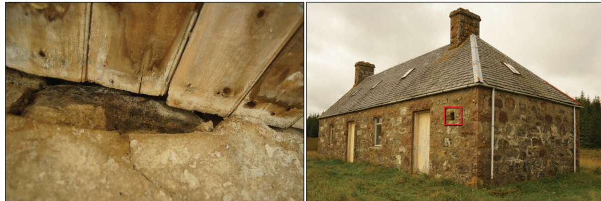
Photo 27. Potential roosting features are gaps between stone walls and timber beams. Photo 28. Bat droppings were found within a ventilation hole on the north aspect of the building (highlighted in red).
