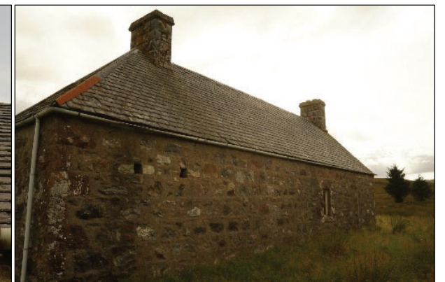
Photo 26. Potential roosting features are gaps under lead flashing and ventilation holes (west aspect).
