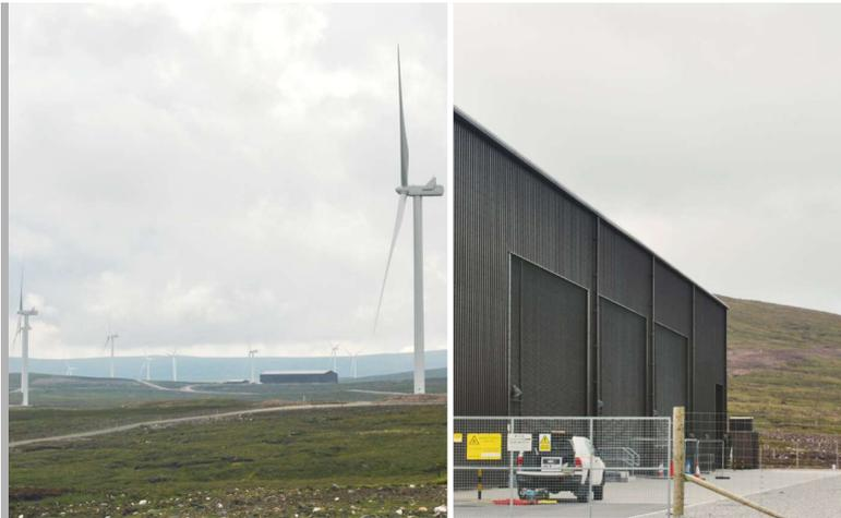
*Buildings would be constructed with a profiled steel cladding and would be likely to appear similar to those for the Stronelairg substation. It is proposed that cladding would be coloured Van Dyke brown, the same colour used for the Stronelairg buildings.*
