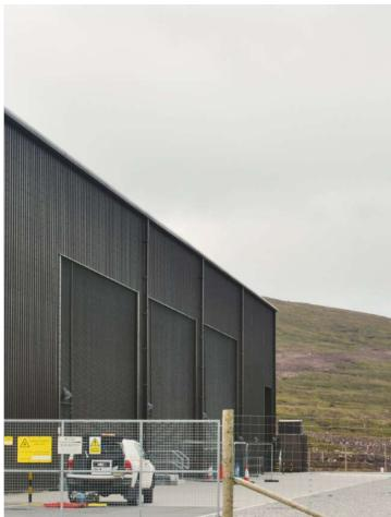
*Buildings would be constructed with a profiled steel cladding and would be likely to appear similar to those for the Stronelaig substation. It is proposed that cladding would be coloured Van Dyke brown, the same colour used for the Stonelaig buildings.*
