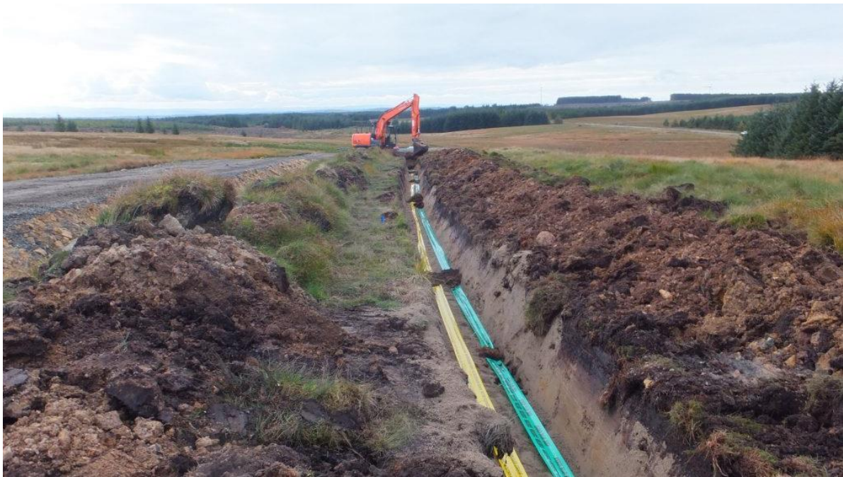
Plate 3: An example photo of a cable being laid using open cut method
