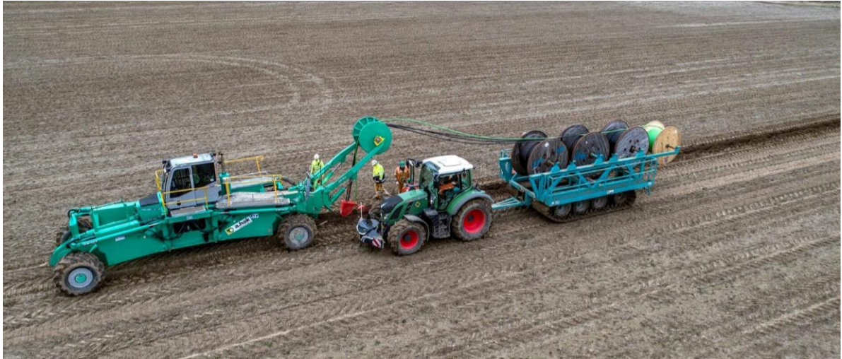
Plate 2: An example photo of cable ploughing
